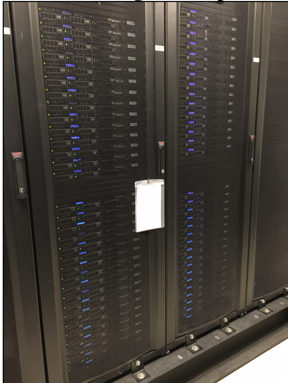
Racks containing 66 compute nodes
