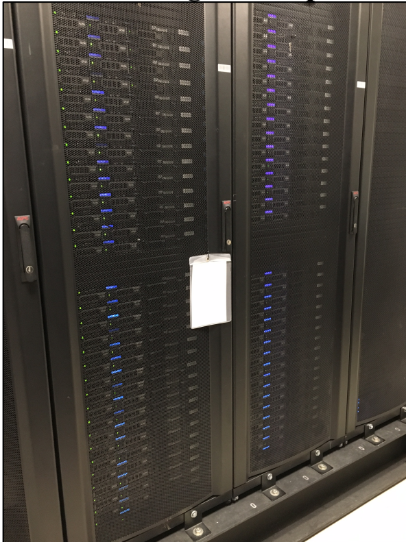
Racks containing 66 compute nodes
