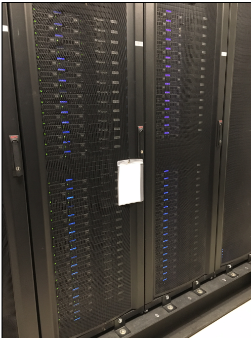
Racks containing 66 compute nodes
