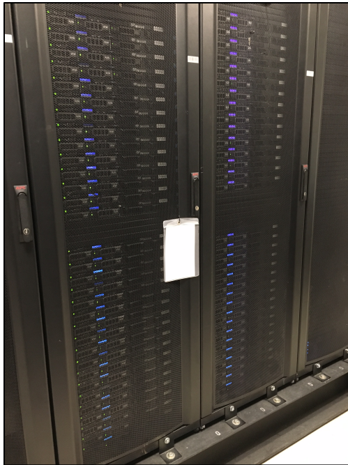
Racks containing 66 compute nodes
